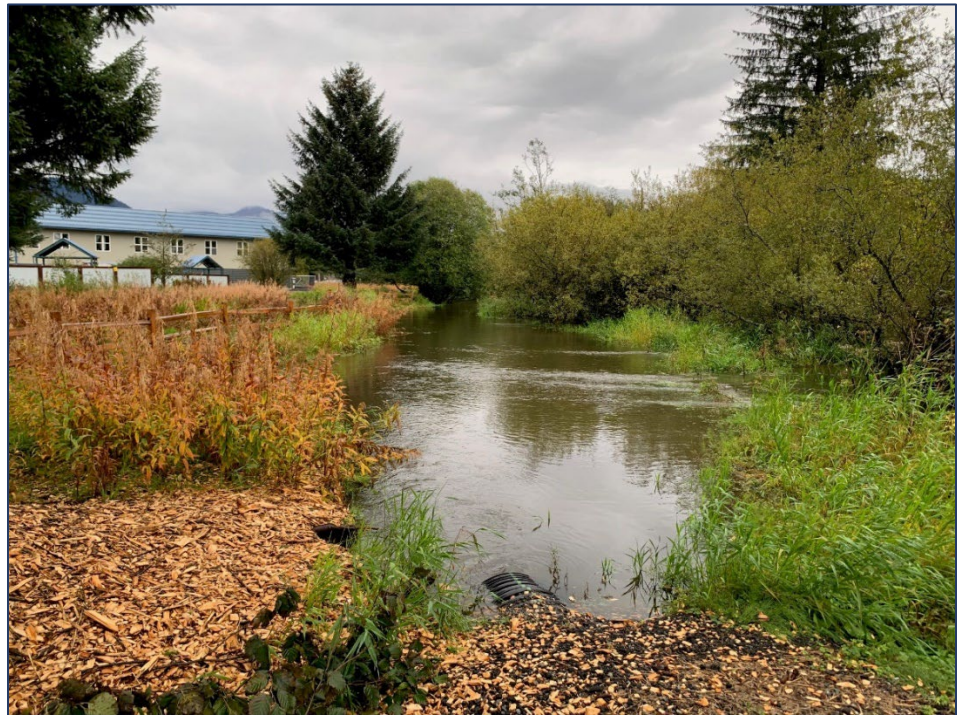
Jordan Creek lower green belt nature-based stormwater infrastructure post installation. Juneau, AK.
