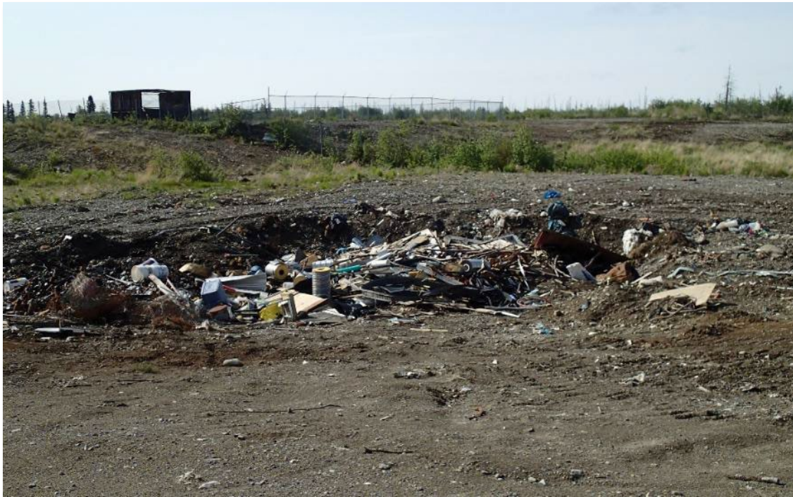
C&D debris disposed of in a trench-and-fill landfill.
