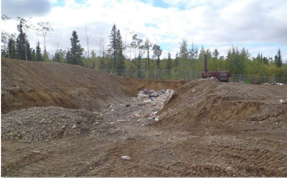
Trench-and-fill working face.
