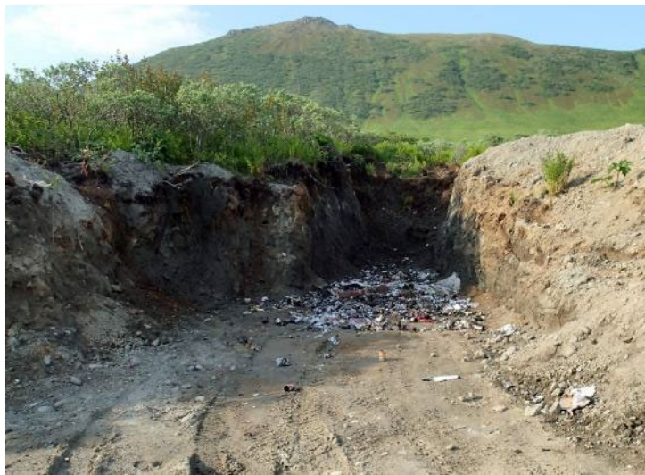
Working face at a trench-and-fill landfill.
