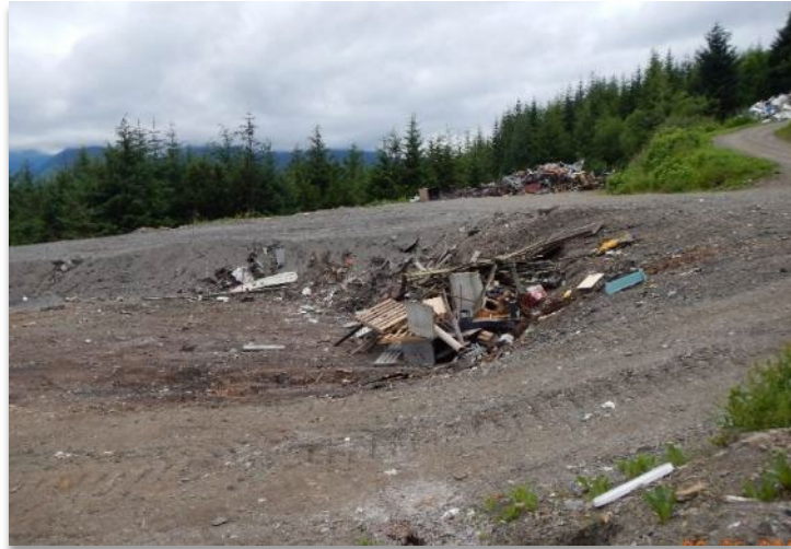
Working face at an area fill.
