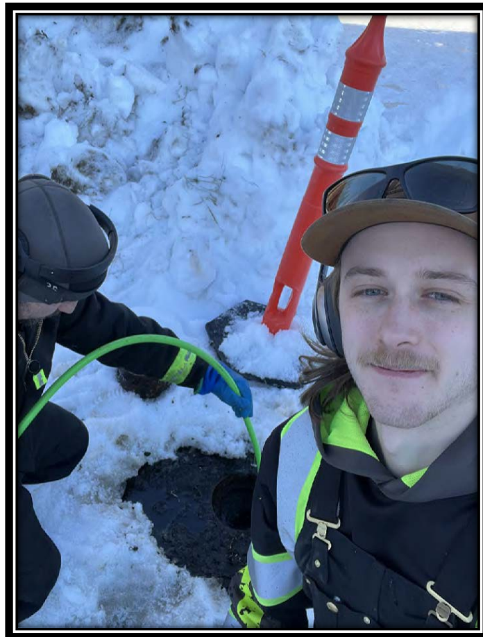
RMW Spencer Singleton assisting the Anderson operator in jetting service lines
