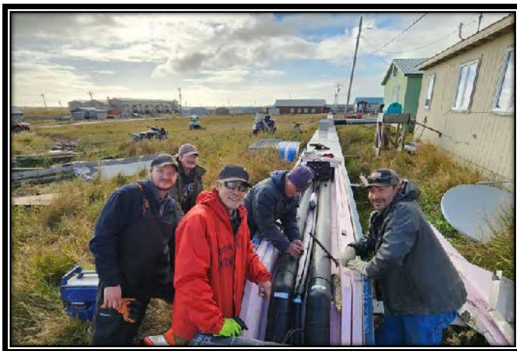
Repairing the glycol line in Hooper Bay
