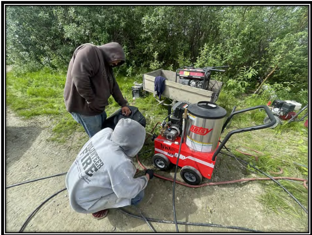
Hooking up the Hosty to have hot water for jetting through the ice in the force main- Kiana Spring 2024.
