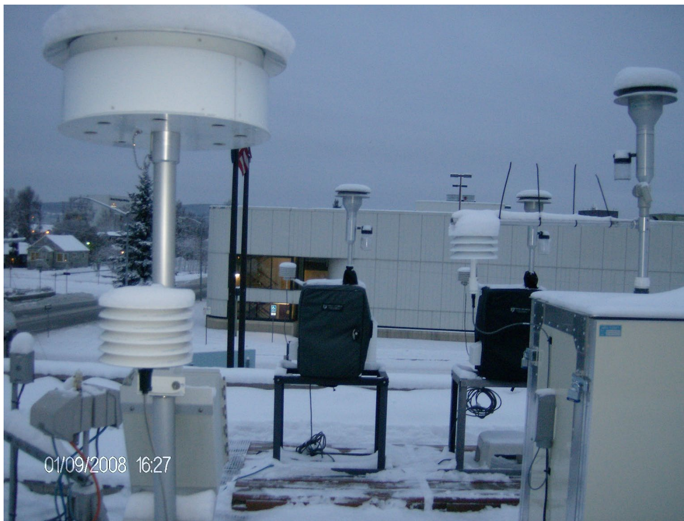
Figure 3 Particulate Matter instrumentation at the FSOB. Photo taken January 9, 2008 looking to the south.
