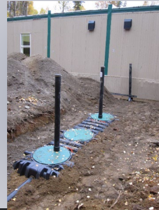
Soil absorption system (treatment and disposal)
