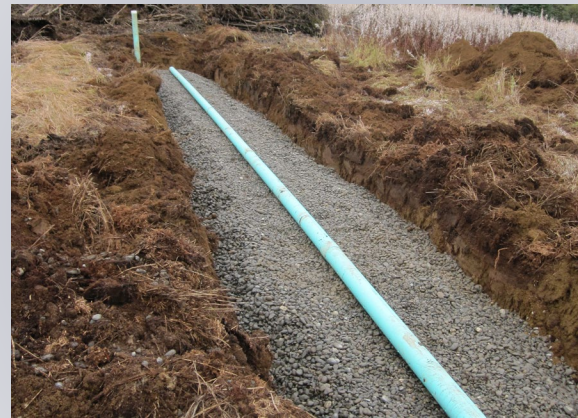
Soil absorption system (treatment and disposal)
