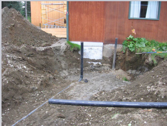
Sewer lines (conveyance system)
