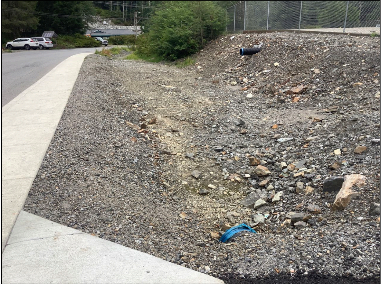
Figure 33. Unvegetated gravel ditch along the south side of Schoenbar road that could be upgraded with check dams, vegetation, and curb cuts to intercept, infiltrate and treat stormwater runoff (biofiltration swale).
