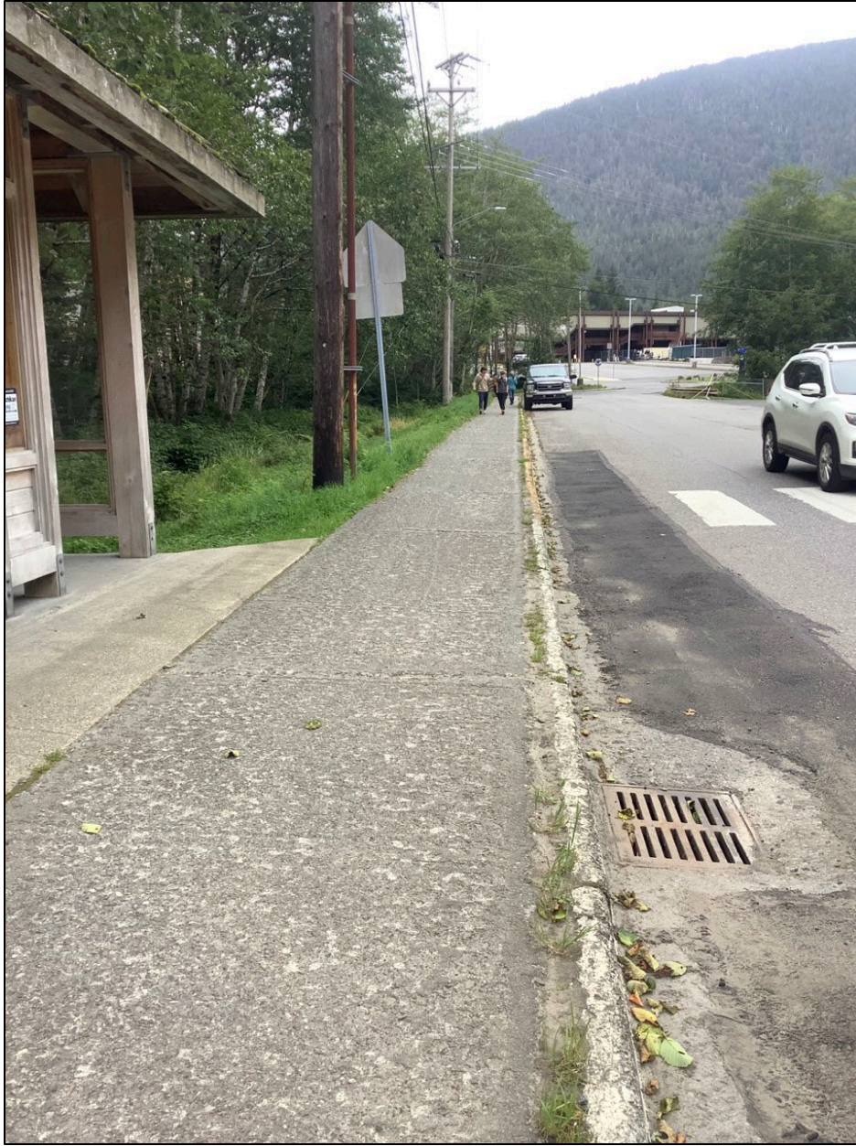
Figure 34. Vegetated buffer on the south side of Schoenbar Rd. that could accept and treat street runoff via curb cuts before it reaches the storm water system. Stormwater treatment capacity of the area could be upgraded with a bioswale or filtration trench.
