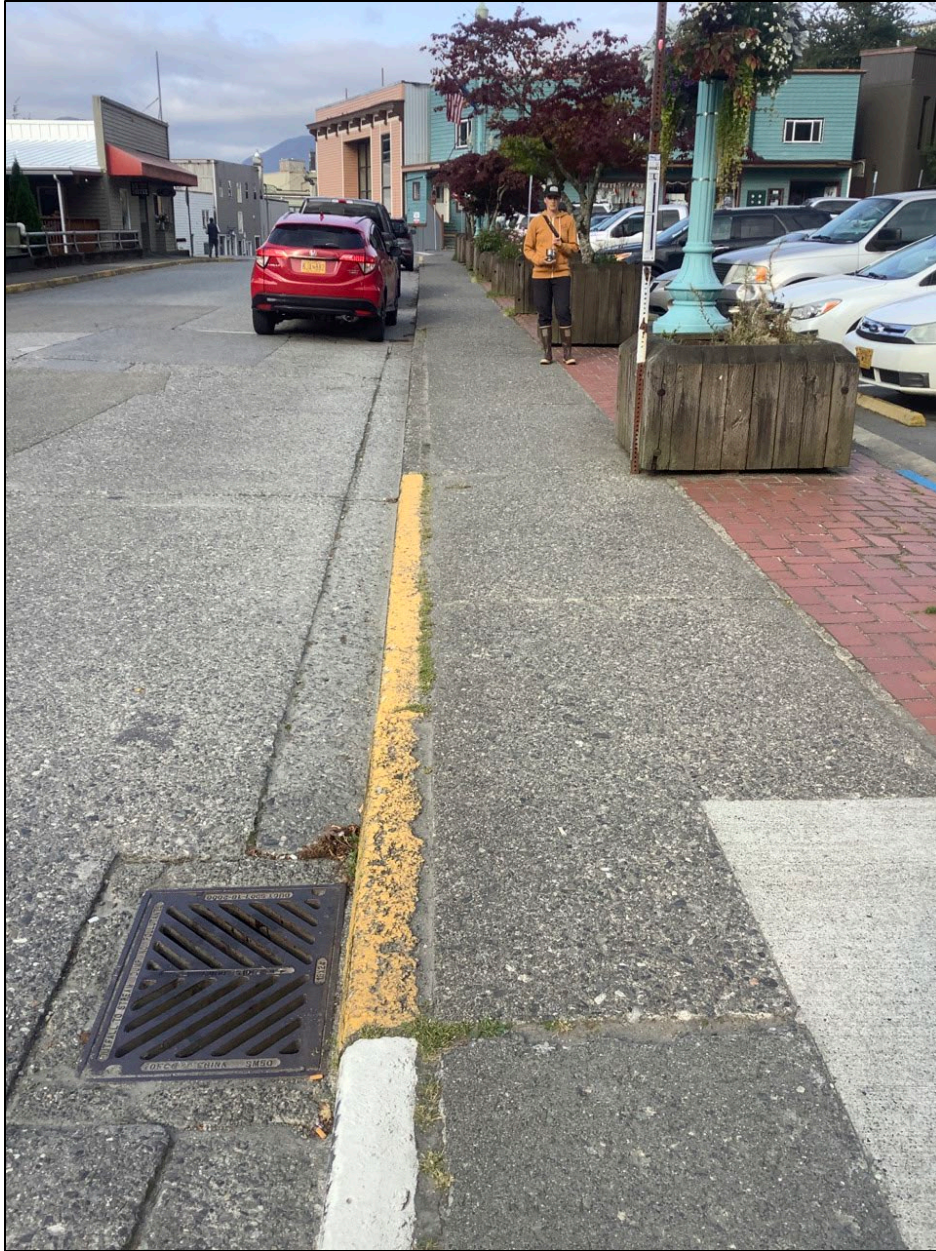
Figure 35. Raised planters on Dock St. that could be converted to bioretention planters that receive and treat runoff from the parking lot and/or street.
