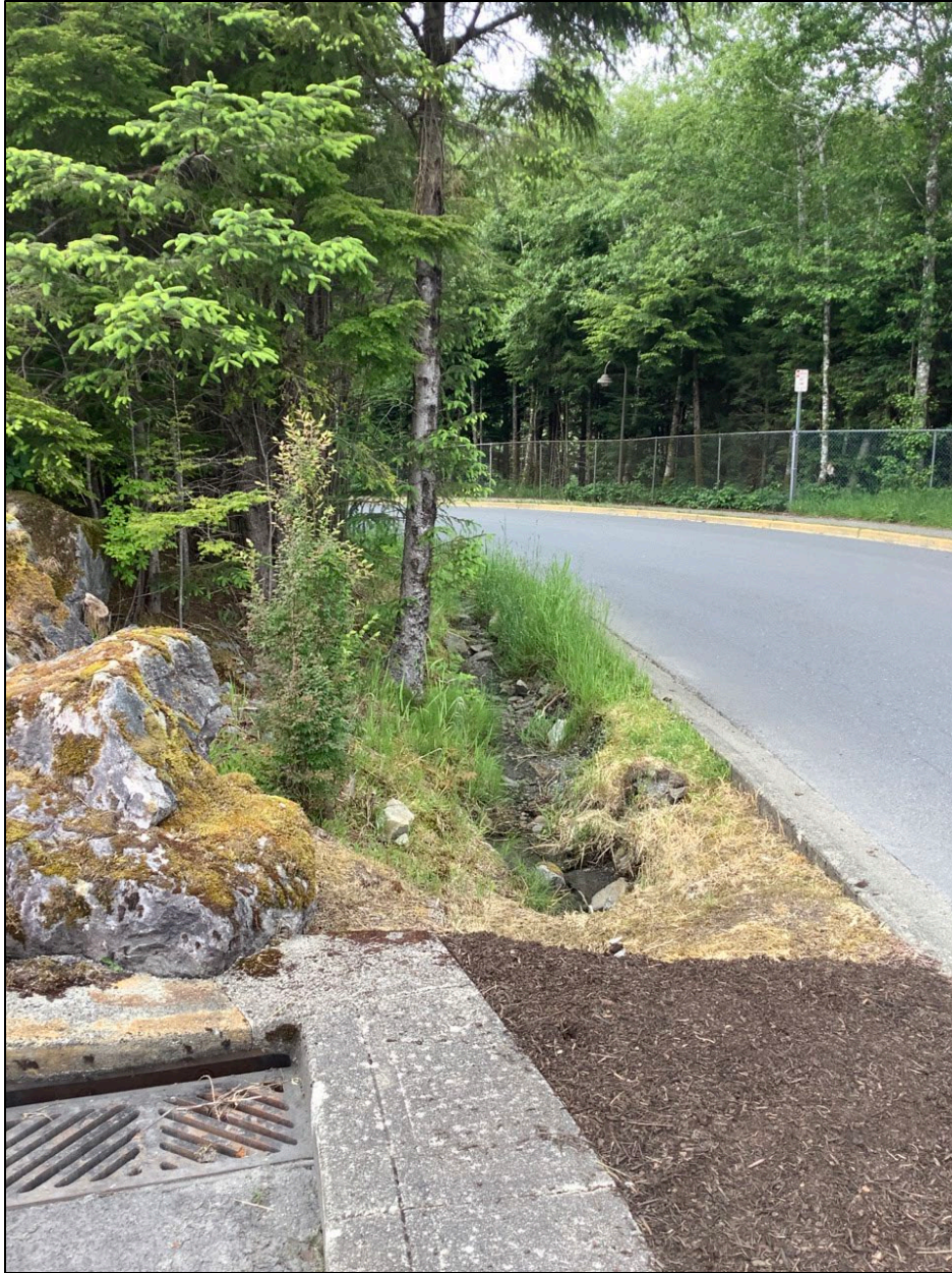
Figure 32. Storm drain at a low point of the Cape Fox Lodge parking lot and the top of a drainage ditch that extends downhill to Park Ave that could be enhanced as a biofiltration swale with check dams and vegetation to promote infiltration and water treatment. Curb cuts could be added to direct more street runoff to the ditch.
