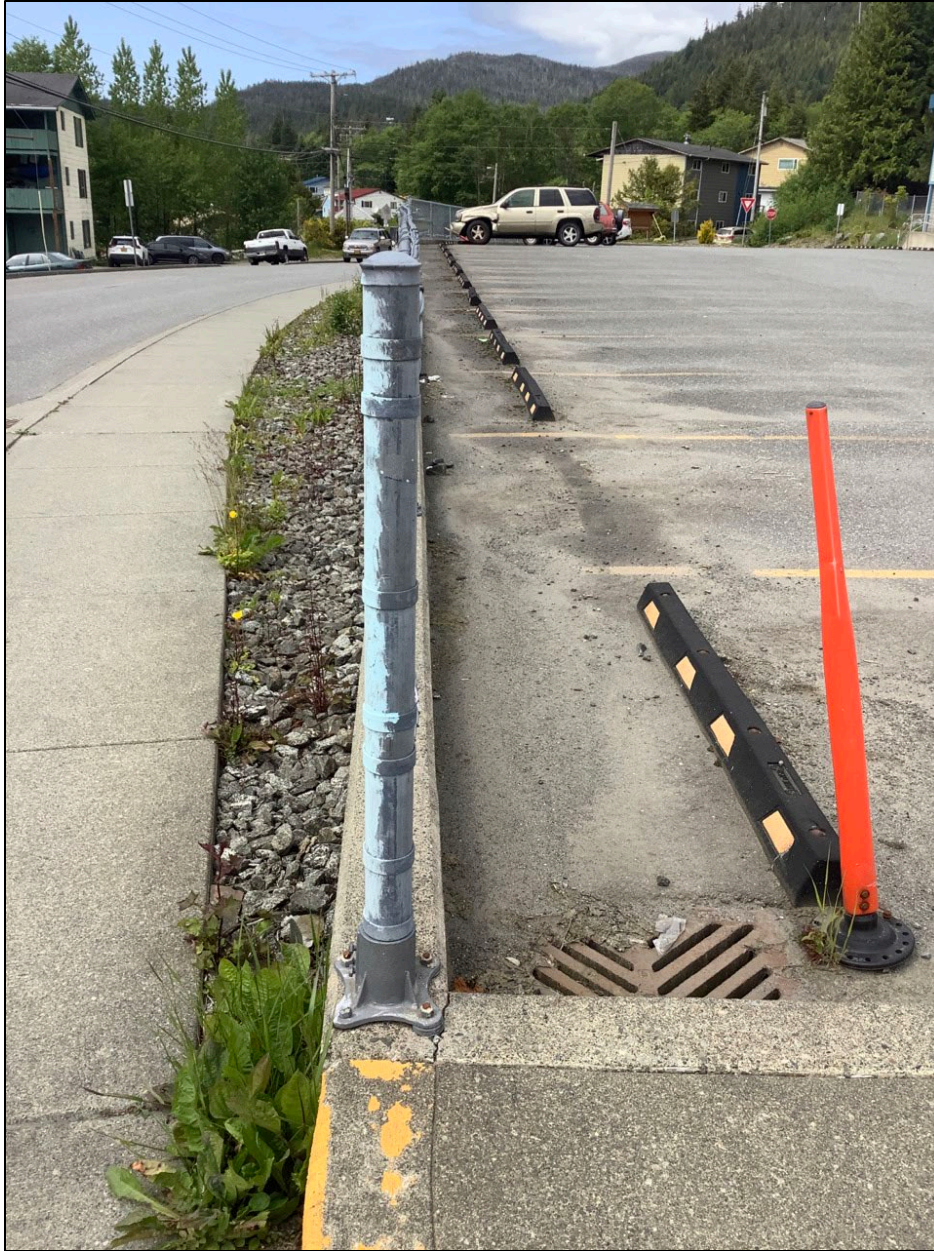
Figure 20. Existing gravel strip in front of Houghtaling Elementary Parking lot. The area could be modified to direct parking lot runoff to the gravel strip for infiltration and treatment before reaching the stormwater system.
