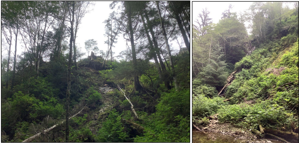
Figure 8. Gullies form on the steep slopes, rapidly transporting stormwater from developed areas on the terrace to the stream. The gully shown in the right photo is below a stormwater outfall.
