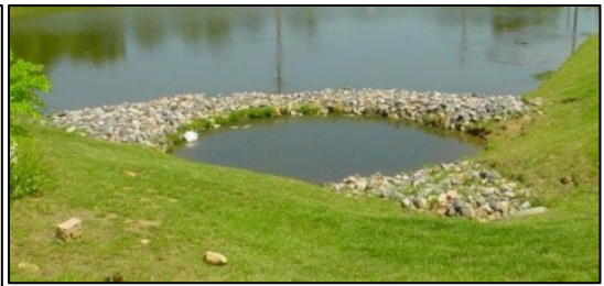
Figure B.1. Examples of pre-treatment facilities: Left: Basic design for an oil-water separator that removes solids and oils (Anderson Waste). Right: A forebay to remove sediment before it enters a retention basin (Massachusetts Clean Water Toolkit).
