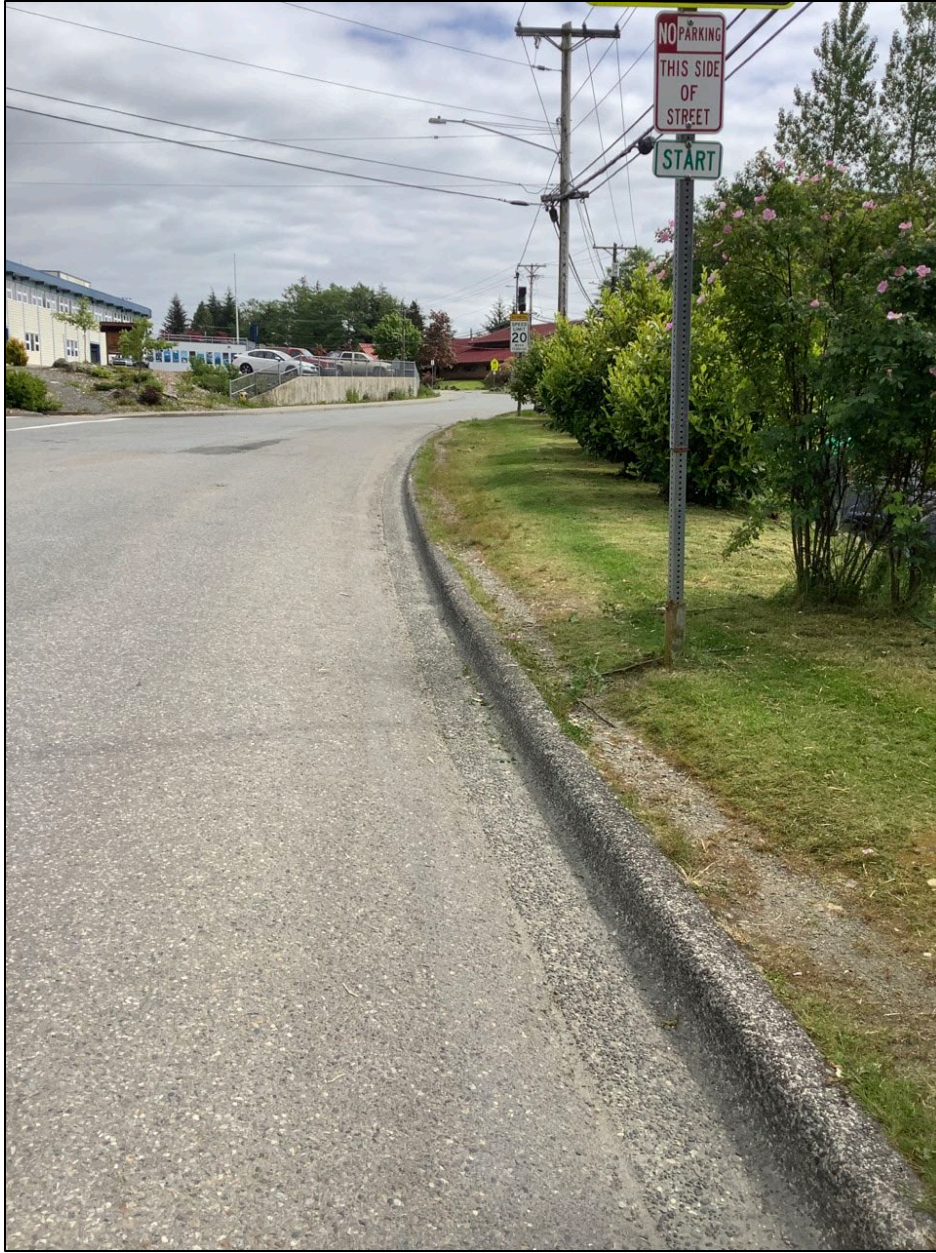
Figure 21. An undeveloped strip of land along Baranof Ave. near Hoadley Creek Crossing that could be modified to accept street runoff before it reaches storm drains. For example, curb cuts and an infiltration basin could be installed.
