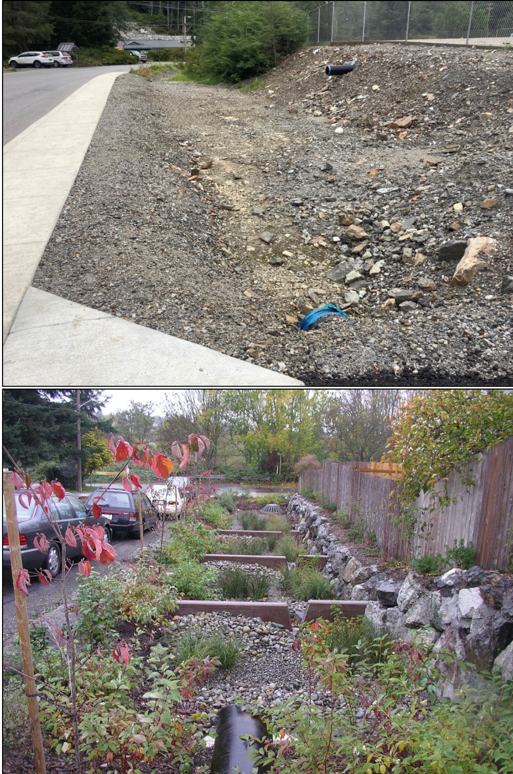
Figure B.3. Top: Unvegetated gravel ditch along the south side of Schoenbar road that could be upgraded with check dams, vegetation, and curb cuts to intercept, infiltrate and treat stormwater runoff. Bottom: Example of a biofiltration swale equipped with check dams to slow water movement from one cell to the next that could replace the gravel conveyance ditch picture above. An elevated overflow drain at the bottom of the feature (upper middle) prevents localized flooding if inflows exceed infiltration capacity.
