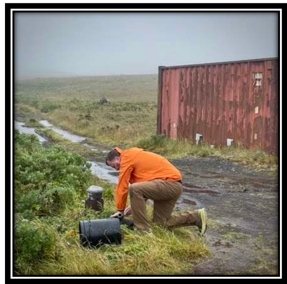
RMW Graber replacing the well cap and seal in St. George
