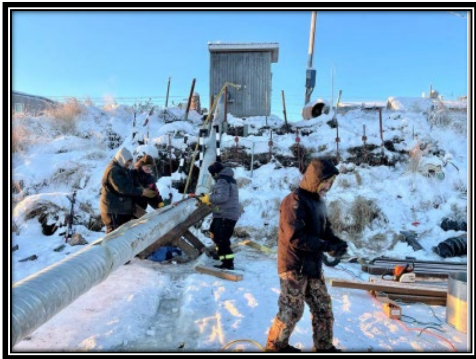
RMW Bruce Nelson with Maniilaq working with Selawik staff to connect a new arctic pipe.
