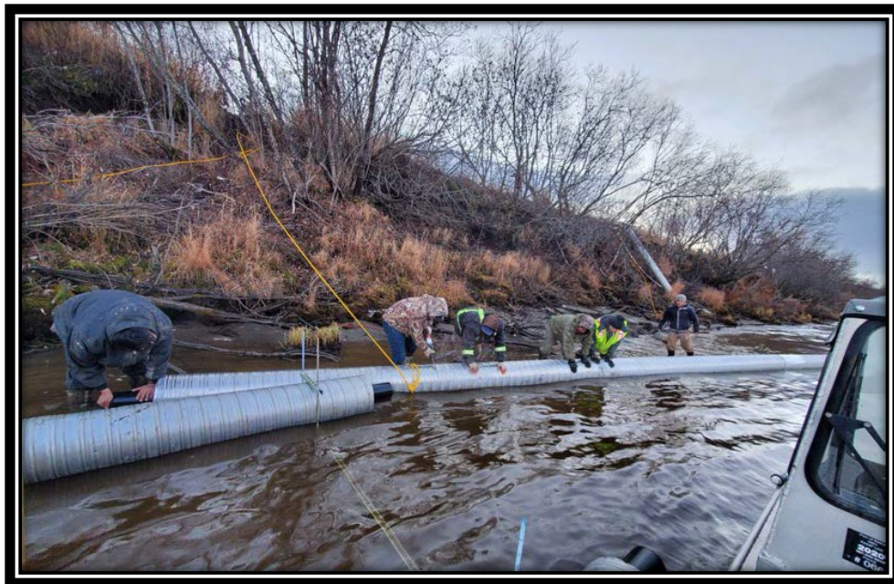
YKHC RMWs assisting with installing arctic piping from the river in Tuluksak
