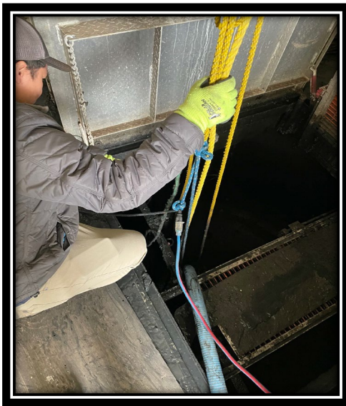
RMW Russell replacing a lift station pump in Nikolai.
