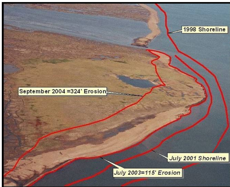
Figure 9-1: Drill Site Erosion
